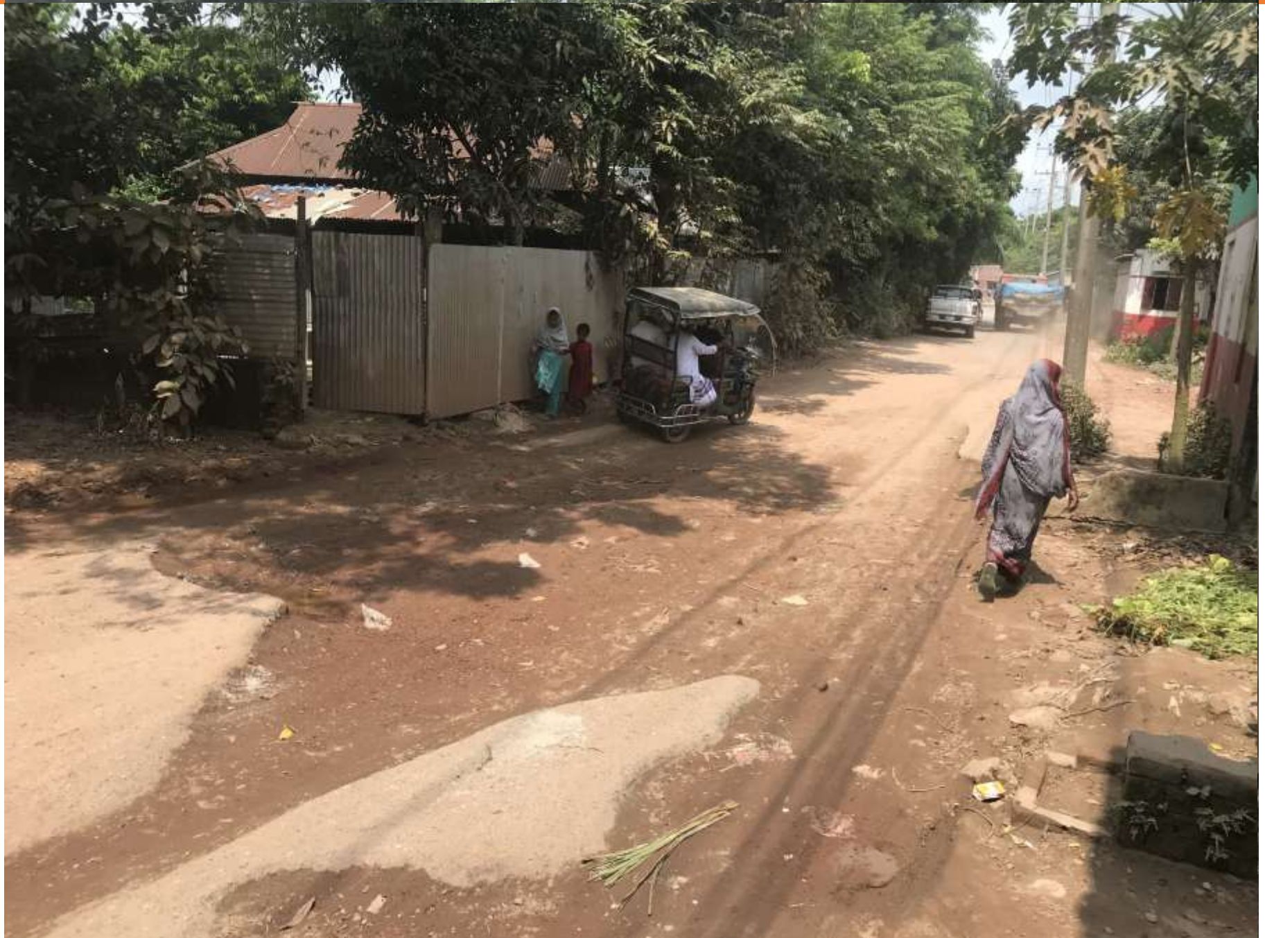
Current Situation of Ruhitpur GC- Baluartack NHW Road (Dharmasur Sonakanda Road)
